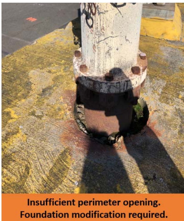
T5 Hydrant Replacement - Extension Perimeter Opening
